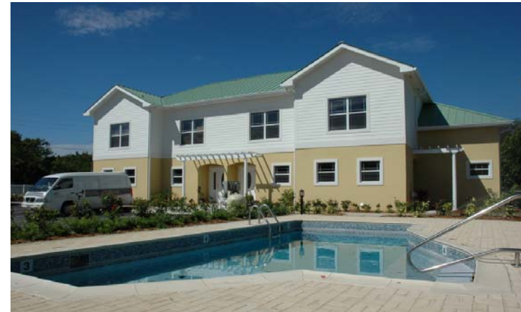
Front elevation over pool to 1 of the 2 buildings
